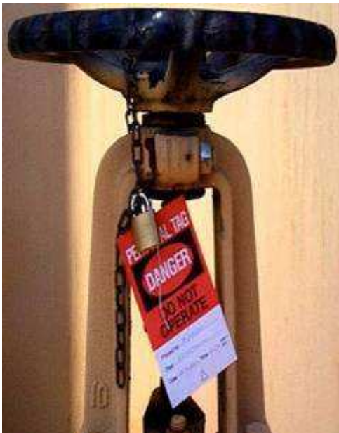
Figure 10. Safe Isolation for Steam Valve
